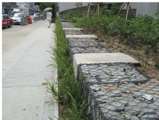
Figure 11 Retention of construction site-hoarding foundations as a feature of the finished retaining wall
