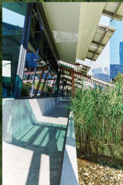
Deep overhangs and trellises on the south facing facade to minimise summer sun penetration
