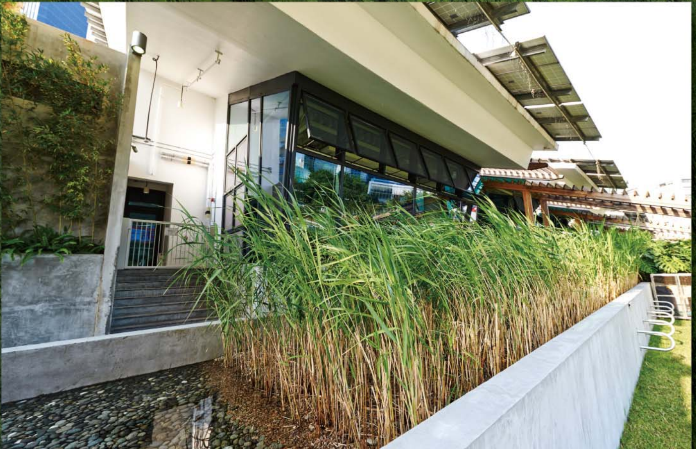
Constructed Wetland system with sub-surface flow to treat grey water and stormwater
