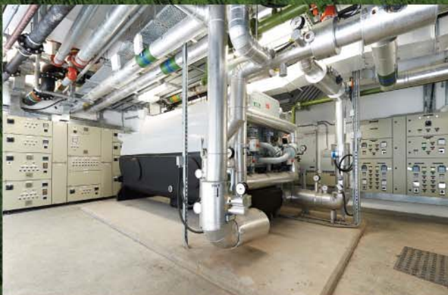
Adsorption chiller driven by recovered heat of the biofuel generator
