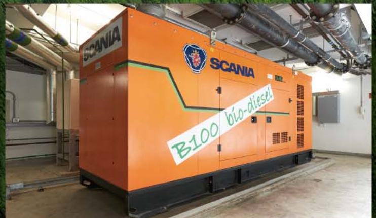
Biofuel tri-generation system uses waste cooking oil for cooling, heat production and power generation
