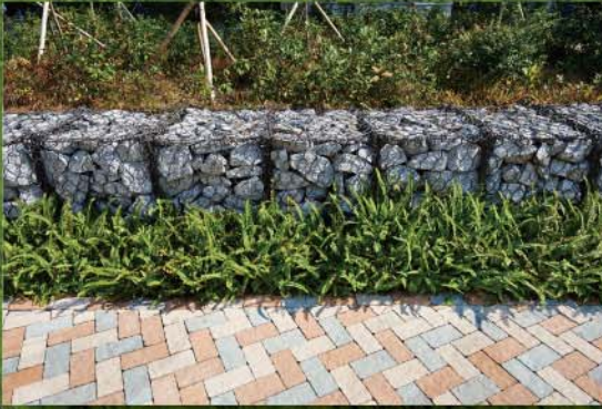
Gabion wall formed from demolition and construction debris
