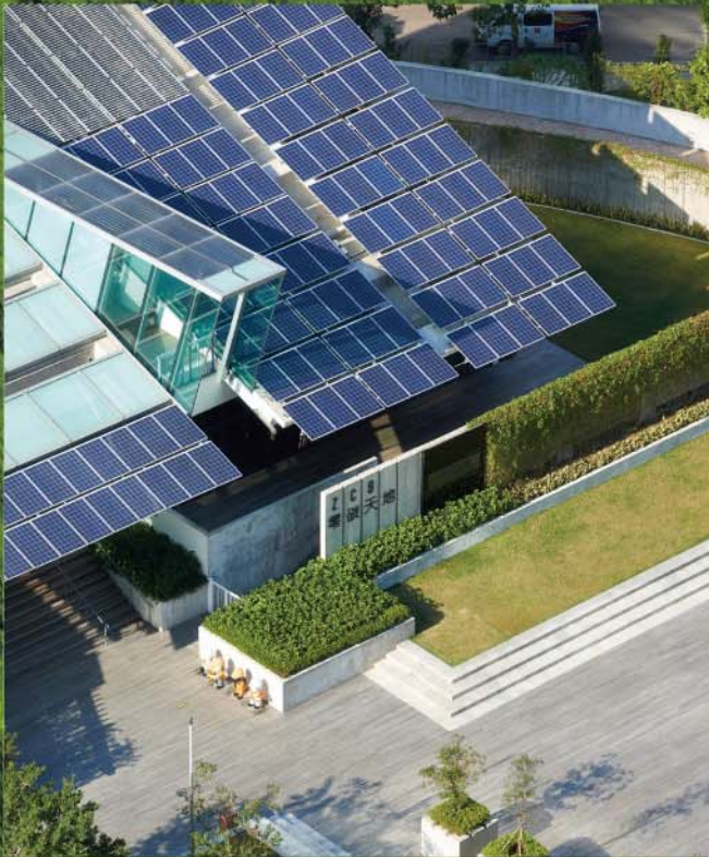
606 polycrystalline photovoltaic panels used on the main roof
