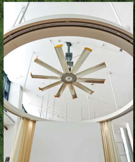
High Volume Low Speed fans move a large amount of air at low speed
