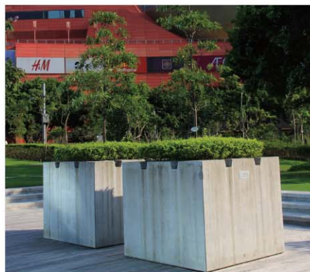
Figure 12 Removable tree planters located above pre-existing drainage culverts
