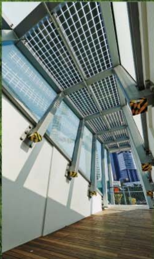
Building Integrated Photovoltaics (BIPV) used as glass roof of the viewing platform
