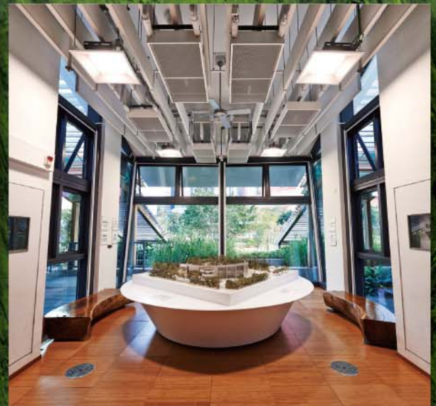
Chilled beams cool occupants via radiant cooling
