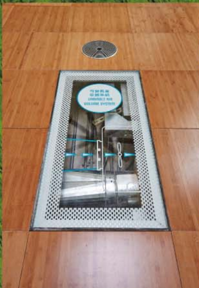
Under floor displacement system cool occupants by convection
