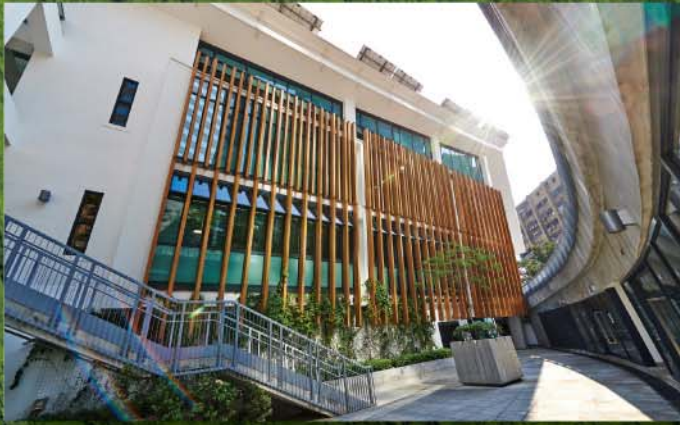
External vertical sunshading fins on northern facade
