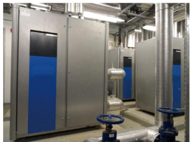
Figure 13 Heat pump
