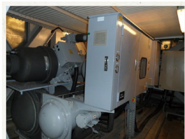
Figure 9 Water cooled variable speed chiller with twin compressors
