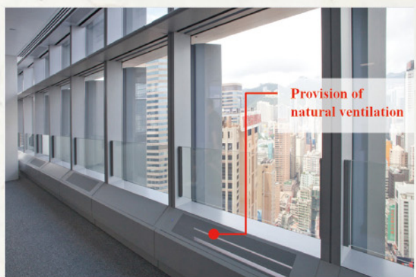
Figure 9 The building combines natural ventilation (via operable vents) and mechanical ventilation/air-conditioning to provide and enhance occupants' comfort and energy efficiency on office floors.
