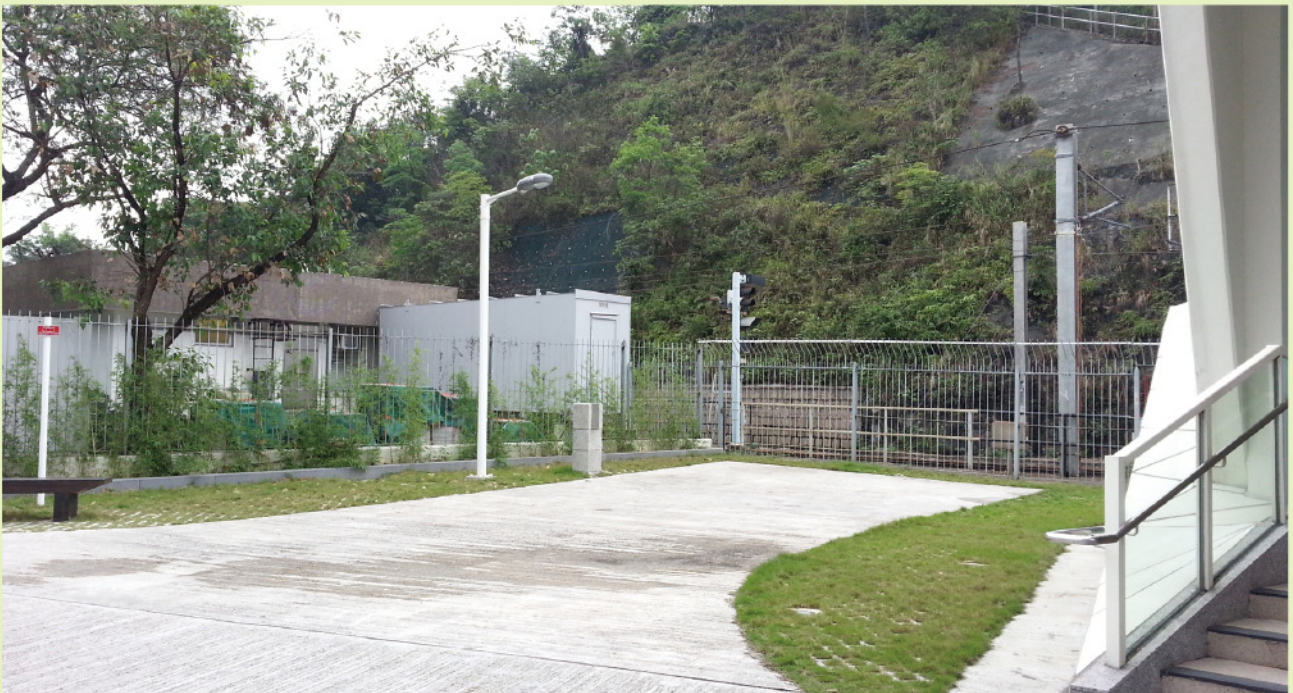
Figure 14 Grasscrete at the sides of the EVA
