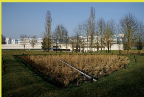
Figure 4 Vegetated ponds for wastewater treatment
