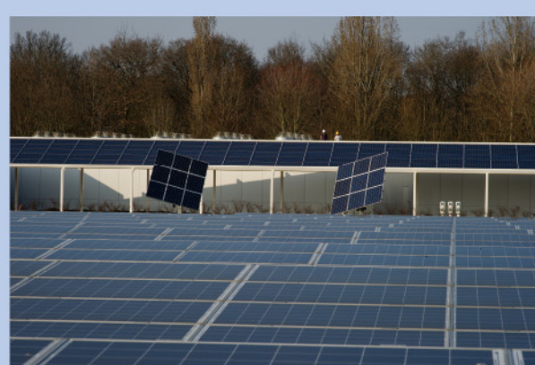
Figure 20 The two trackers – one is fixed and one is actively tracking the sun
