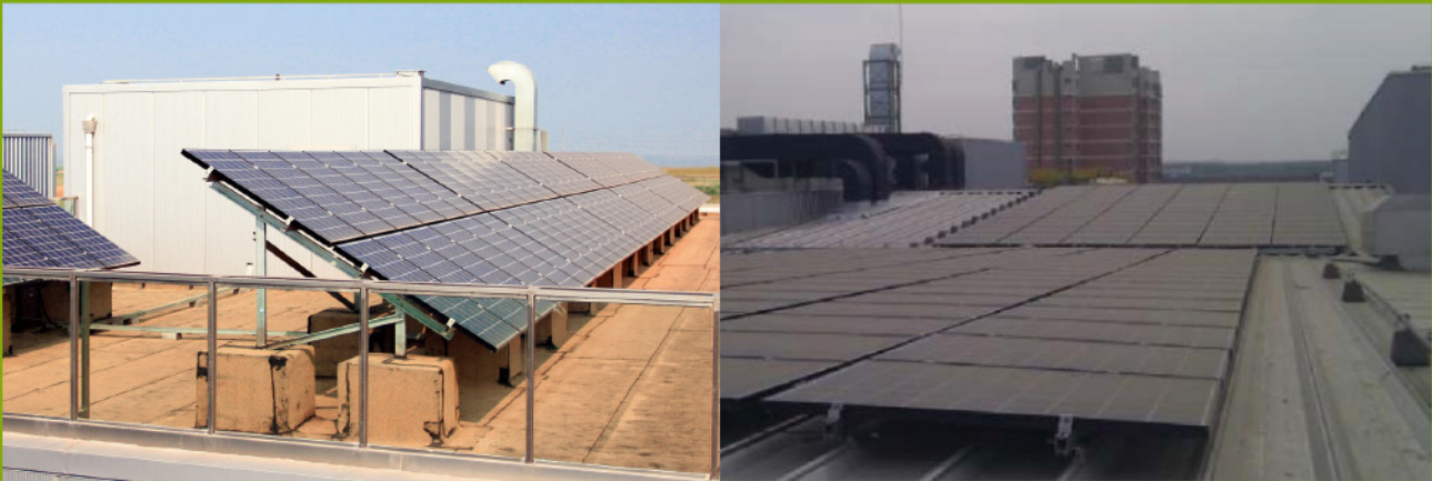
Figure 12 Roof top solar photovoltaic application
