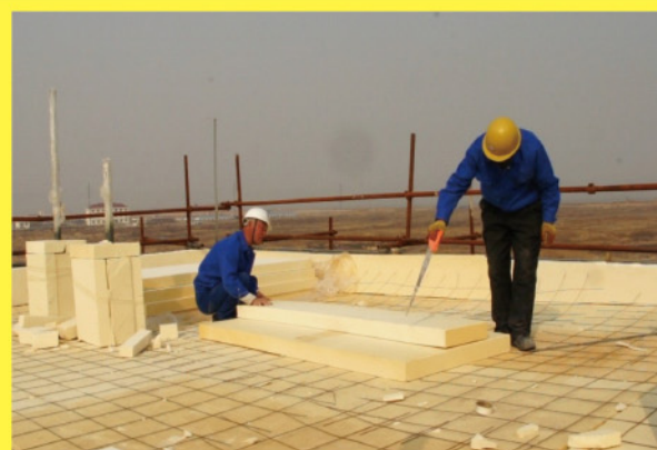
Figure 11 Roofing insulation application
