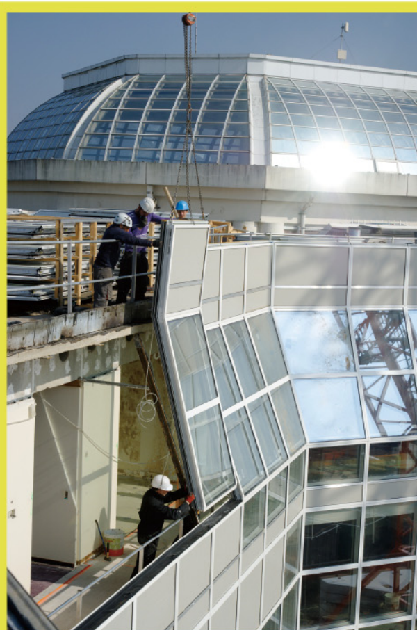
Figure 16 Installation of the double skin façade
