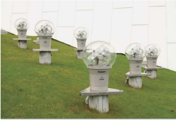
Figure 12 Solar tracking light pipes maximise sunlight collection by use of automatic solar tracking devices
