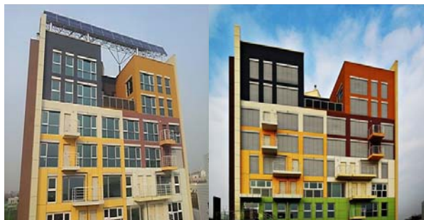
Figure 22 External venetian blinds on ZCGH: opened (left) and closed (right)
