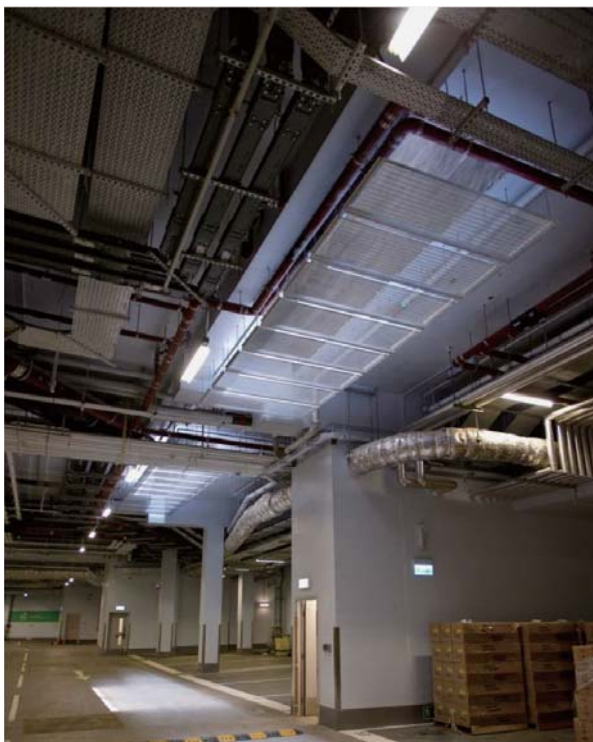
Figure 8 Solar chimney in the basement carpark
