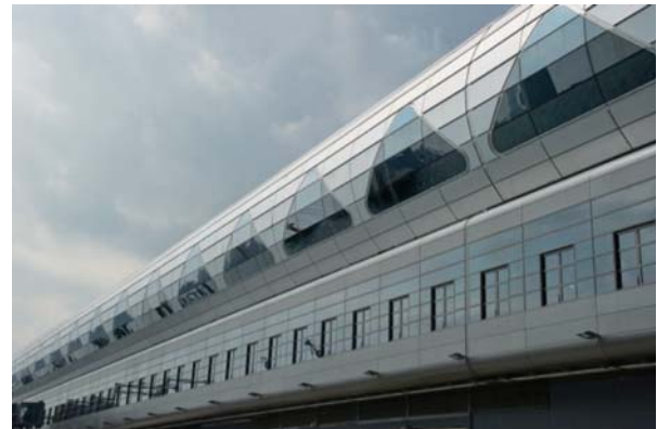
Figure 6 The glazing is conical and triangulated in shape. The wide base of the glazing allows maximum visibility for passengers with the top portion pointed to limit overall solar heat gain
