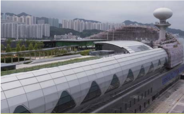
Figure 7 Elements of the building envelope were carefully selected to attain an Overall Thermal Transfer Value (OTTV) not exceeding 18\text{W/m}^2 , therefore, heat transfer through the building envelope is kept to a minimum
