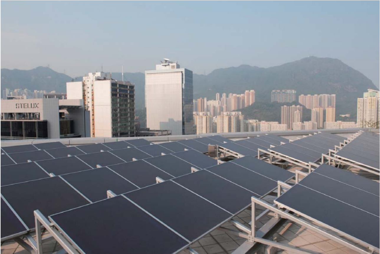
Figure 15 Solar PV Array on at Roof Level
