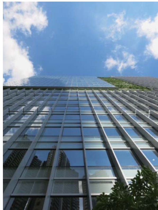
Figure 7 Application of sunshades to reduce heat gain and glare
