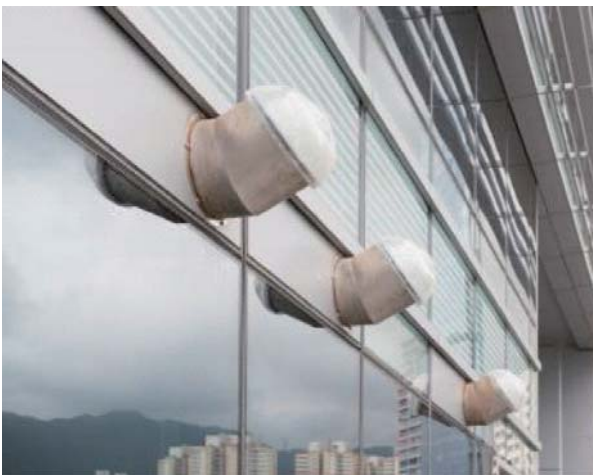
Figure 13 Anidolic light in the façade for building management office
