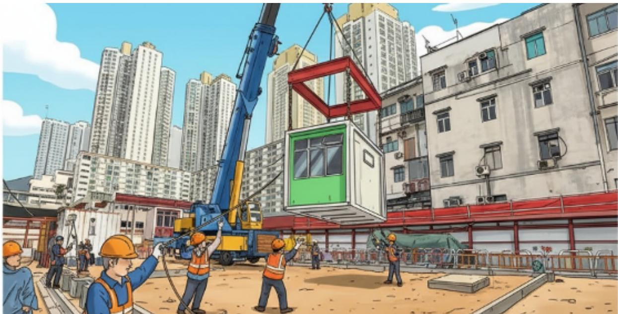
Modular Integrated Construction (MiC) is an innovative building method similar to stacking blocks, where prefabricated small components are assembled together to form a building.
